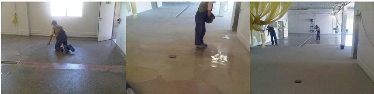
Installing the membrane
