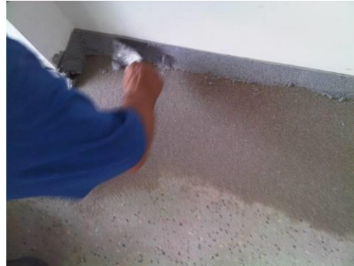
Installing the cove
