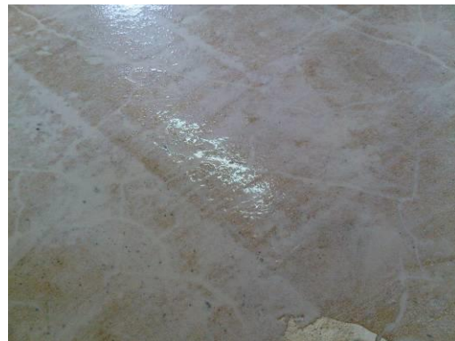
Cracks are sealed with Plastifloor® 510
