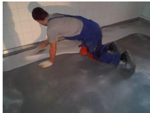
Installation of the coating
