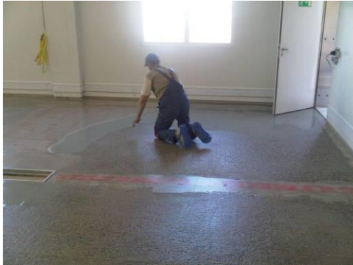
Installing the membrane
