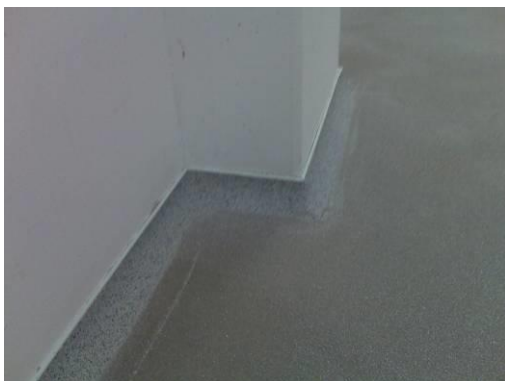
Connection to the wall with membrane
