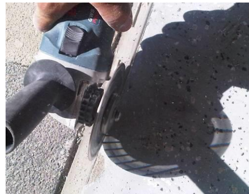
Junctions are being cut in
