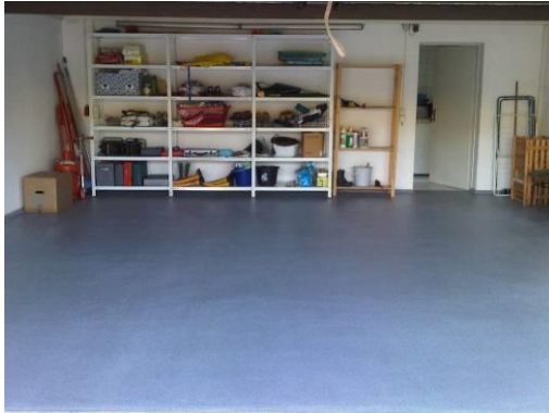
The finished garage floor .
