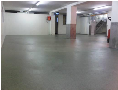
The finished floor on Sunday evening.
