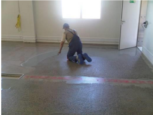
Installing the membrane
