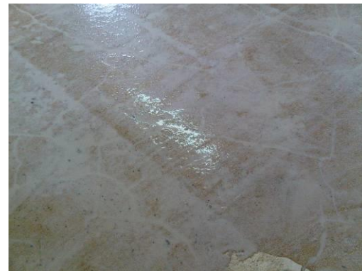
Cracks are being cast with Plastifloor® 332 + PET
