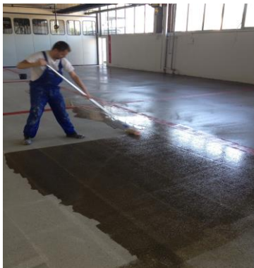
Application of primer Plastifloor® 112
