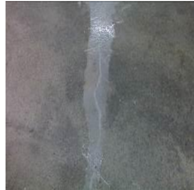
Cracks were sealed
