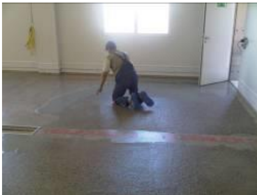
Installing the membrane
