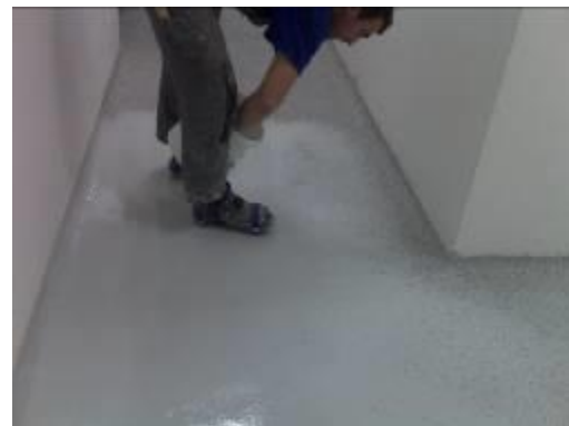
Broadcasting the top coat with colour flakes
