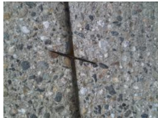
Joints are being cramped
