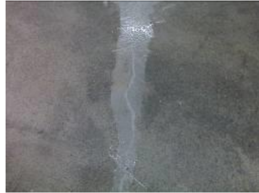
Cracks are being cast with Plastifloor® 510 + s/l filler
