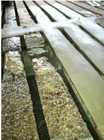
Concrete repair with Plastifloor® acrylic resin mortar.
