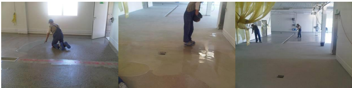
Installing the membrane
