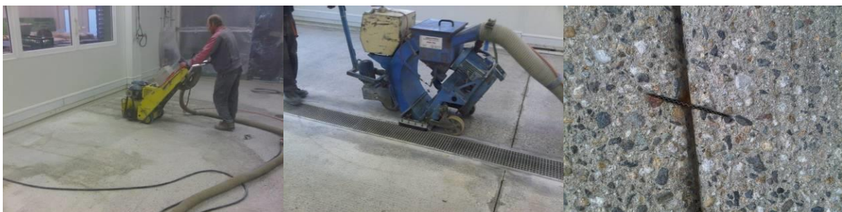
Milling off the EP coating
