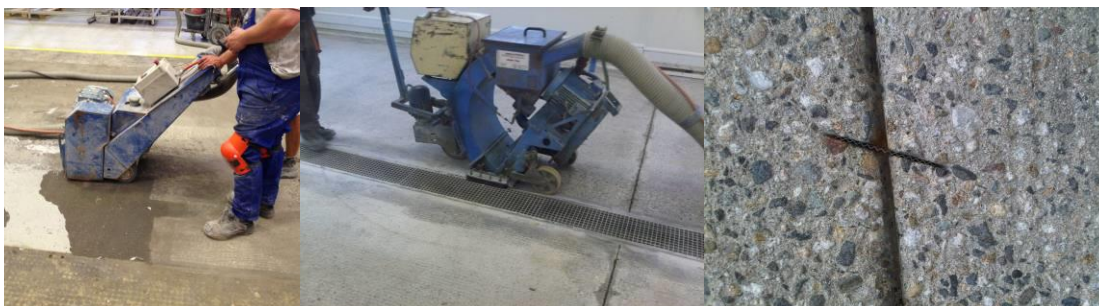
Milling off the EP coating
