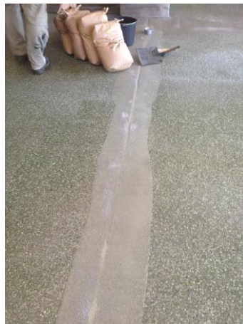
Joints where filled with Plastifloor® 9332 + s/IPET (1:1)
