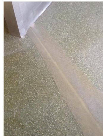
Joints where filled with Plastifloor® 9332 + s/IPET (1:1)
