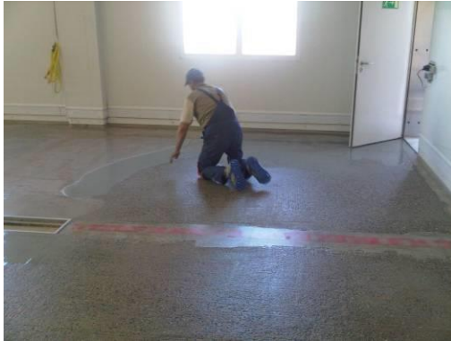
Installing the membrane
