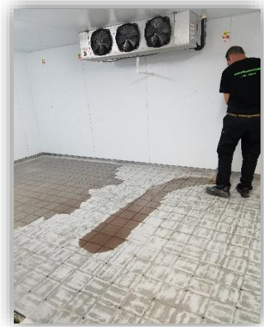
9. Priming the whole area with roller 'lamb skin'
