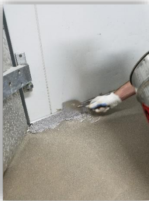
16. Pre-primed substrate and slightly broadcasted
