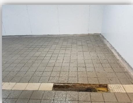
10. Holes need to be filled with mortar
