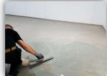
15. Applied with Swedish trowel
