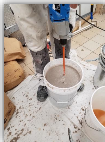
11. Mix Plastifloor® 510 with mix C2 and Hardener
