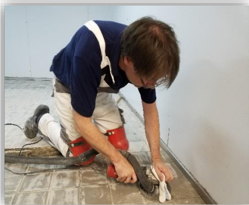
1. Grinding the Substrate
