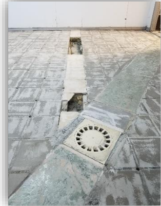
3. Substrate ready for priming
