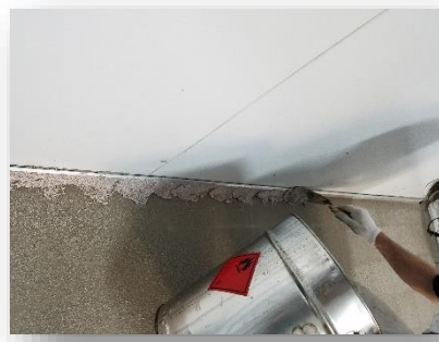
17. Use spatula to equally spread the mixture
