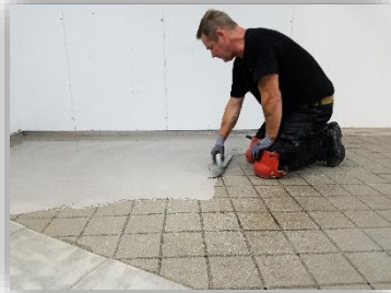
13. Applying membrane Plastifloor® 332
