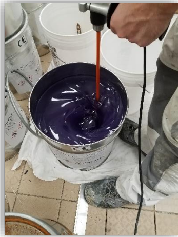
7. Mixing Plastifloor®112 with Hardener 50W
